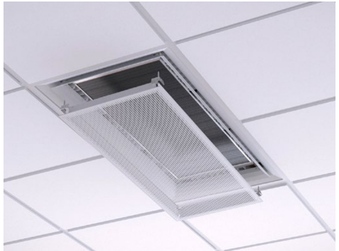
Figure 12. Removing the face plate to access the coil
