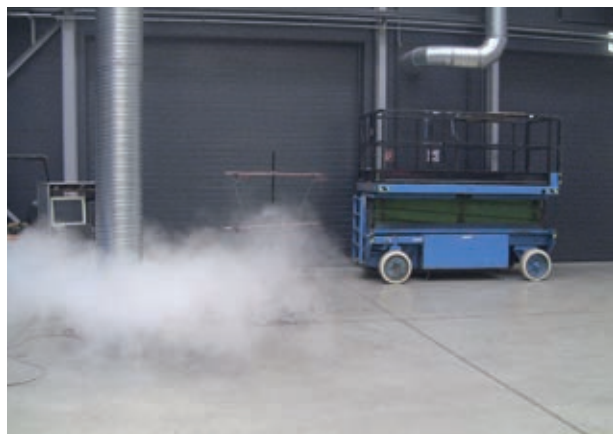
Fig. 14: Circular displacement outlet positioned on the floor
