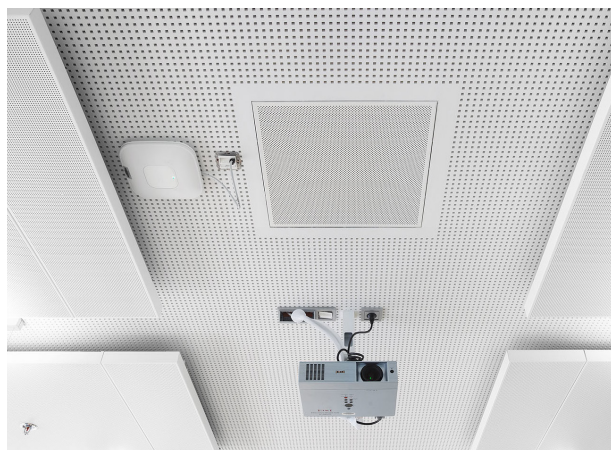
Fig. 8: Opticlean installed in a perforated gypsum plasterboard ceiling
