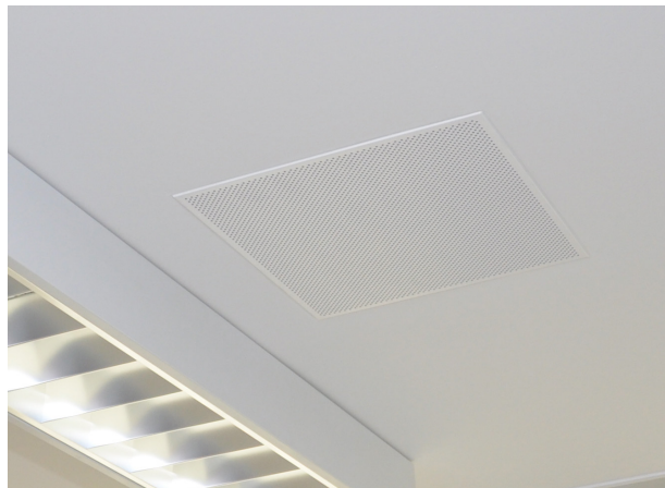
Fig. 7: Opticlean installed in a gypsum plasterboard ceiling
